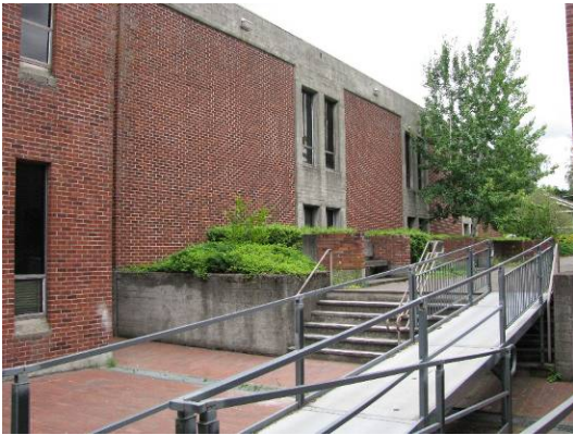
Classroom addition (213D), looking east.
