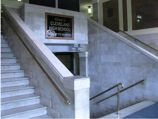
Main entrance and stairwell (213A).
