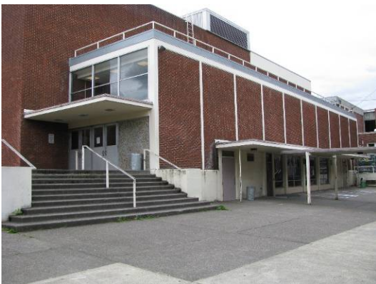
Entrance to new gymnasium (213B), looking Northeast.
